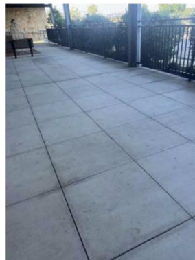
FOL Patio and Handicap Ramp Pressure Washed
