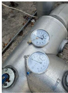
Old Chiller Pump Gauges
