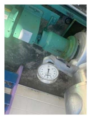
Installed Old Chiller Pump Gauge to New Pump
