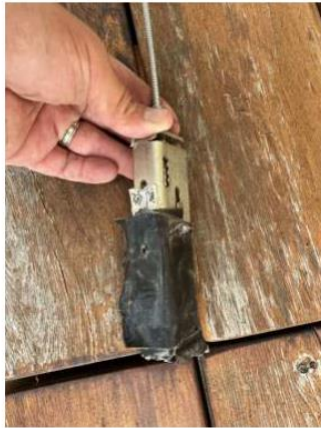
Alert Lock & Key Repaired Broken Exit Cable On Childrens Patio Door
