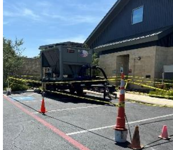
Temporary Chiller Installed Until New Is Delivered
